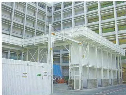
Workers' hard work paid off. The scaffolding was completed.
