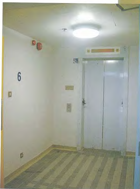
Lift in the new building
